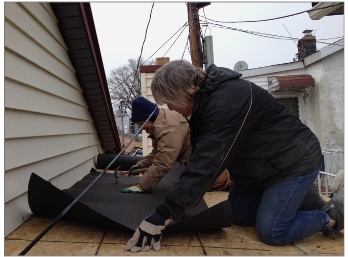
Nancy J. and Janet roofing one of the bungalows.
