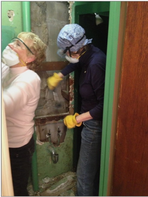
Nancy Y. and Suzanne demolish a bathroom.
