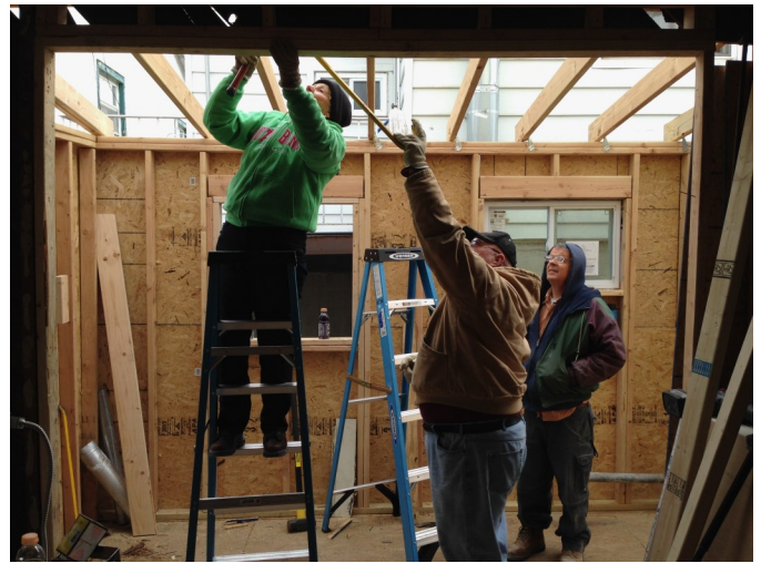
Preparing the roof.
