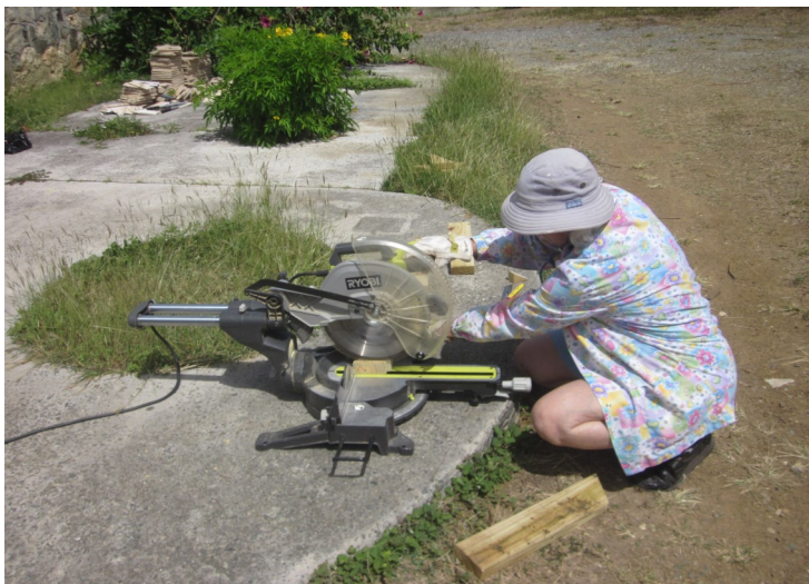
Janet cutting purlins with chop saw
