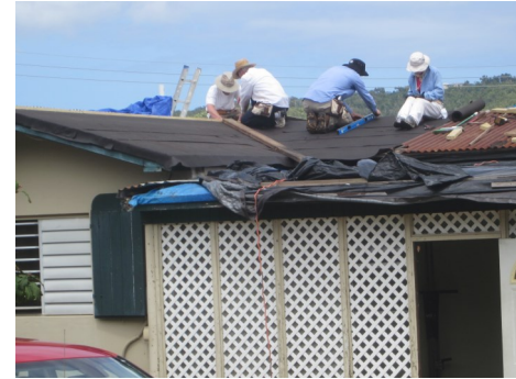
Re-felting of roof
